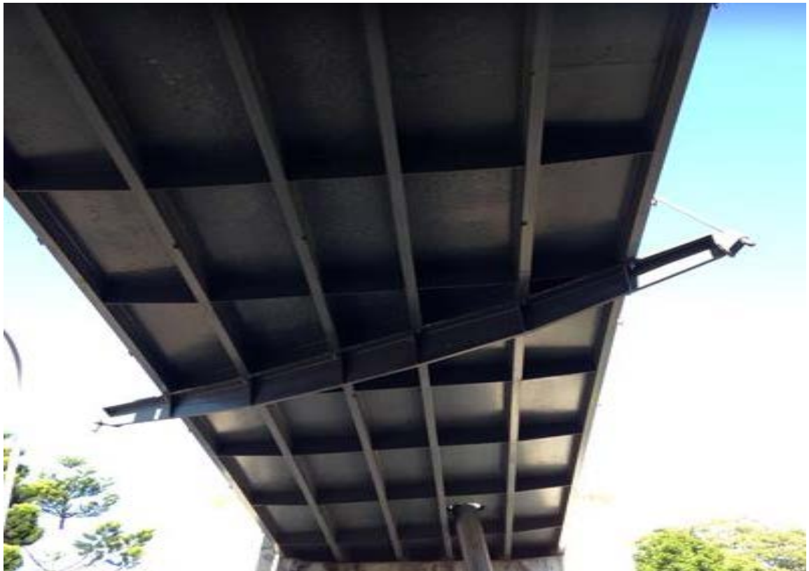
Underside of bridge to be cleaned and repainted
