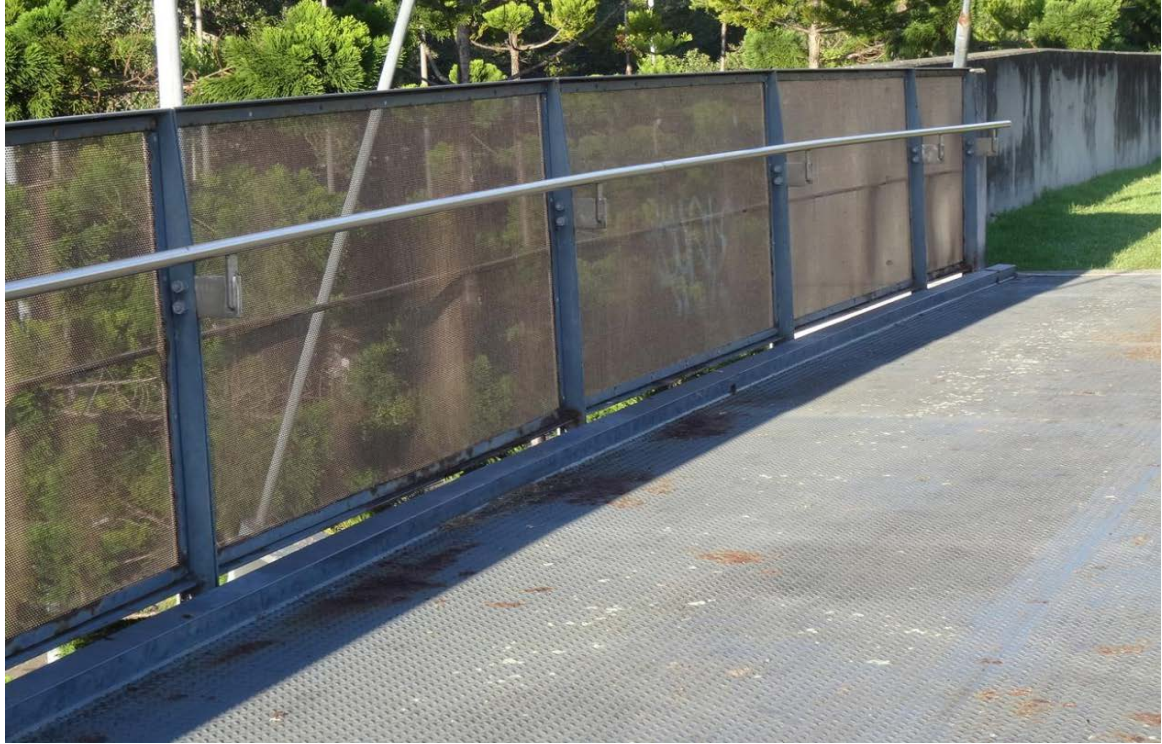
Fence to be removed, repainted and reinstalled
